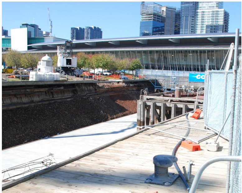
Duke and Orrs Dock, 9 April 2009 - new floor and side work, old side timber with old POLLY wharf. (L. Rex)
