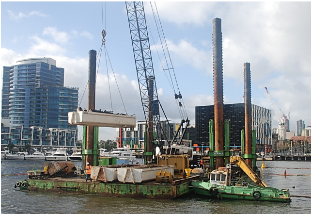
The end of Lady Chelmsford: The jackup barge with grab and crane together with the transport barge, bins and workboats at Central Pier berth 14. A full bin is being moved from jackup barge to transport barge. Materials were transported to North Wharf for loading on to trucks. (Image L. Rex).
